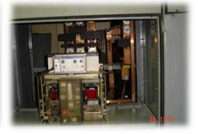
Cable laying and panel terminations and installation of 3000A change over switch at Indomie Otta, Ogun State
